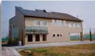
Super Eco House in Ota City, Gunma Pref. completed in 2006
