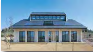
Super Eco House in Ota City, Gunma Pref. completed in 2010
